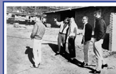
Zeta members view new house under construction
